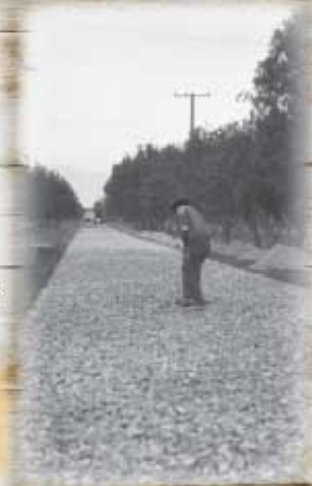
Paving on Hammer Ave.
