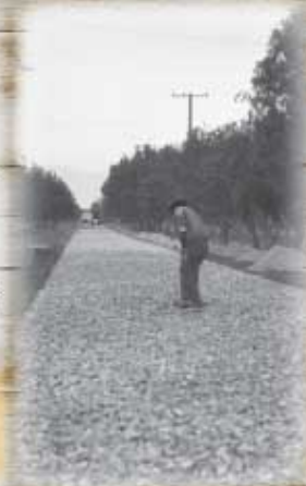
Paving on Hammer Ave.
